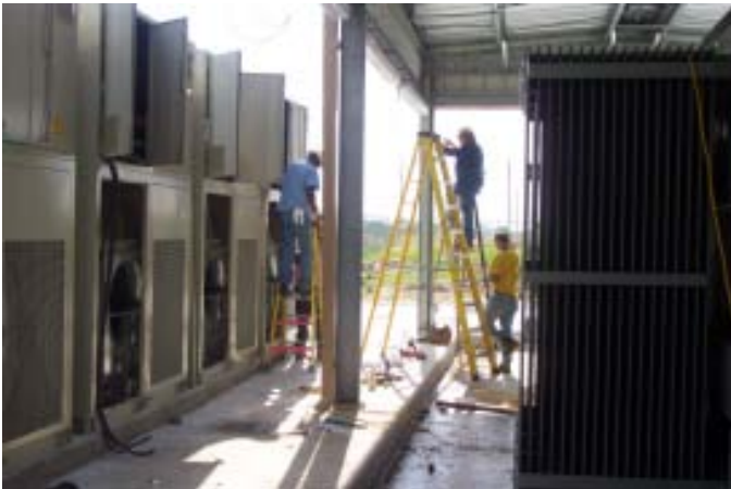
Switchgear Installation
