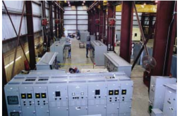
Switchgear and Controls Manufacturing Plant Assembly Bay
