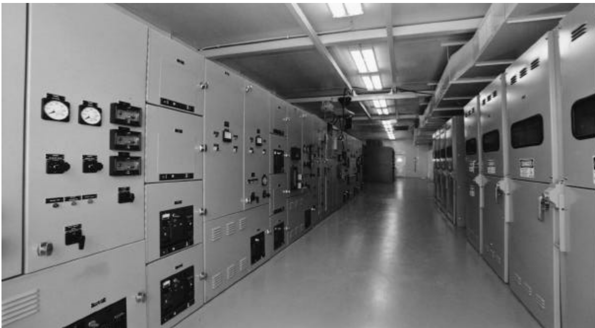
Figure 2—Interior view of type ISB Building
