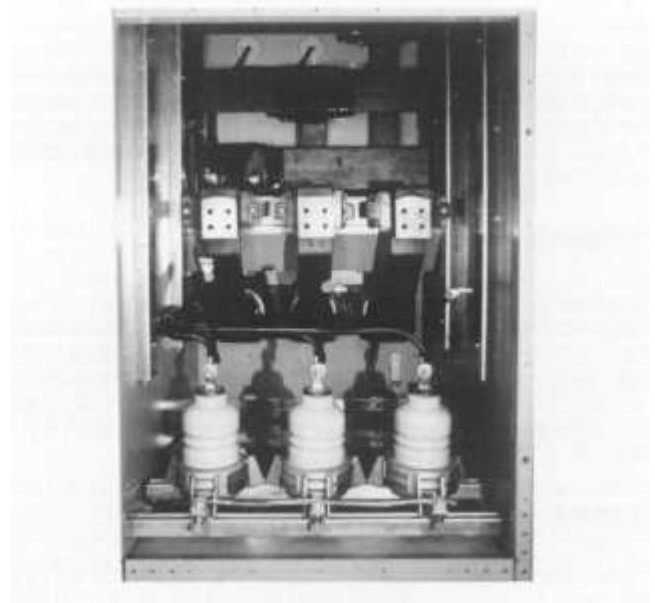
Main Bus—Note: Barriers removed for photo
