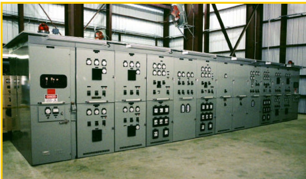
6.6KV Generator Control & Distribution Switchgear
