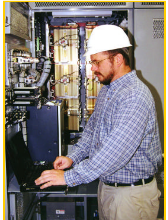
Calibration of Digital Controls for SCR Unit
