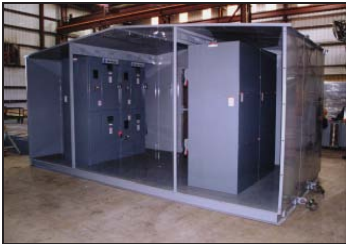
Add on to existing 5KV substation
