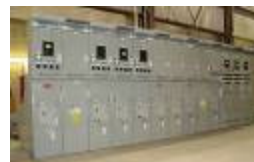
Medium-voltage 11KV IEC Generator control and distribution switchgear built for Boeing SBX project
