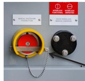
Mechanical through door trip with breaker lock-out
