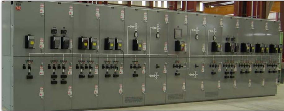
**27kV Two High Switchgear**
